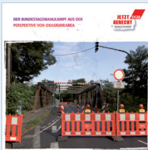
Brücke in Duisburg/Moers
